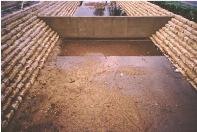
**Description:** Multi-chamber structure designed to treat stormwater runoff through filtration, using a sediment forebay, a sand bed as its primary filter media and an underdrain collection system (typically).
