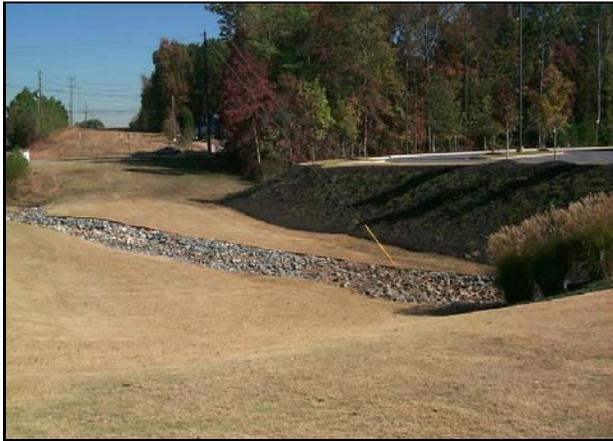
**Description:** A surface storage basin or facility designed to provide water quantity control and limited water quality benefits through detention and/or extended detention of stormwater runoff.
