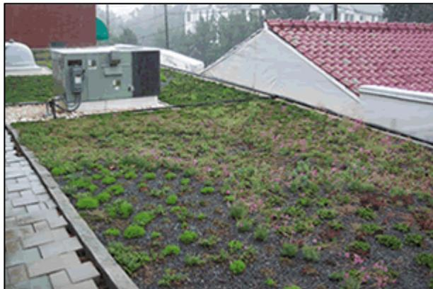
**Description:** A vegetated roof cover composed of hardy plants growing in an engineered plant medium, filter cloth, drainage layer, and waterproofing membrane. Greenroofs provide benefits such as reducing runoff volume and peak discharge rate, reducing building cooling costs, and prolonging roof life.
