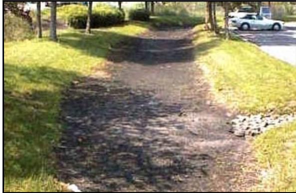
**Description:** Excavated trench filled with stone aggregate used to capture and allow infiltration of stormwater runoff into the surrounding soils from the bottom and sides of the trench.
