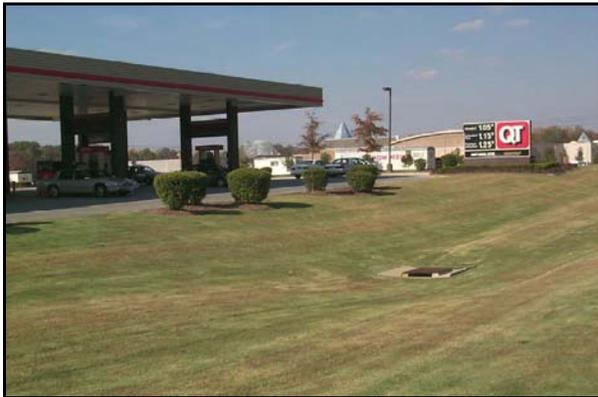
**Description:** Uniformly graded section of land that is densely vegetated and is designed to treat runoff through vegetative filtering and infiltration. Water enters the filter strip along its width and runs across the length of the filter strip.
