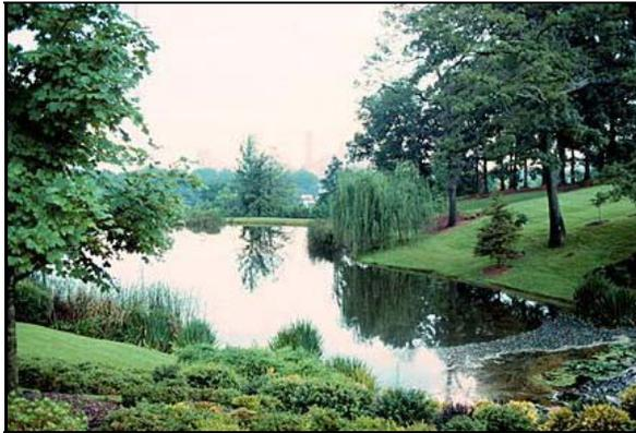
**Description:** Constructed stormwater detention basin that has a permanent pool (or micropool). Runoff from each rain event is captured and treated in the pool primarily through settling and biological uptake mechanisms.
