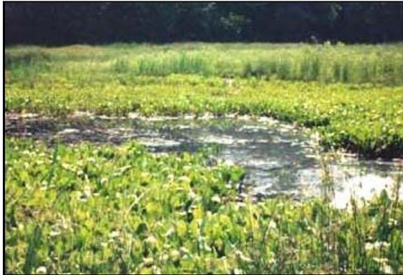
**Description:** Constructed wetland systems that are designed specifically for the purpose of managing stormwater. Runoff volume is stored and pollutants are removed in the wetland facility.
