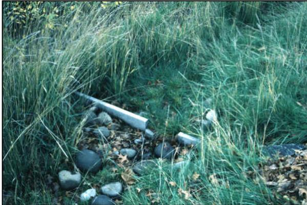
**Description:** Vegetated open channels that are designed to capture and treat stormwater runoff within dry or wet cells formed by check dams or other methods.
