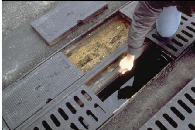
**Description:** Multi-chamber structure designed to treat stormwater runoff through filtration, using a sediment forebay, a sand bed as its primary filter media and an underdrain collection system (usually). Perimeter sand filters are located along the edge of impervious areas.
