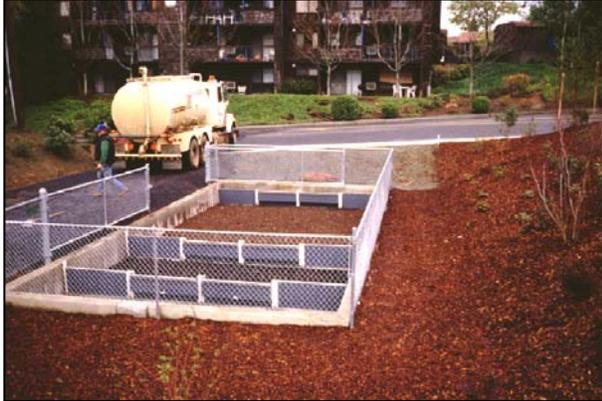
**Description:** Usually a two chambered stormwater treatment practice and variant on a sand filter. The first chamber is for settling and the second is a filter bed of organic media. Large particles settle out in the first chamber and finer particles and other pollutants are removed in the second chamber.
